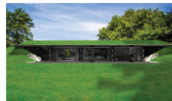
«Earth sheltered home» maison passive - Nathalia Australie Arch. : Baldwin O'Bryan architect
